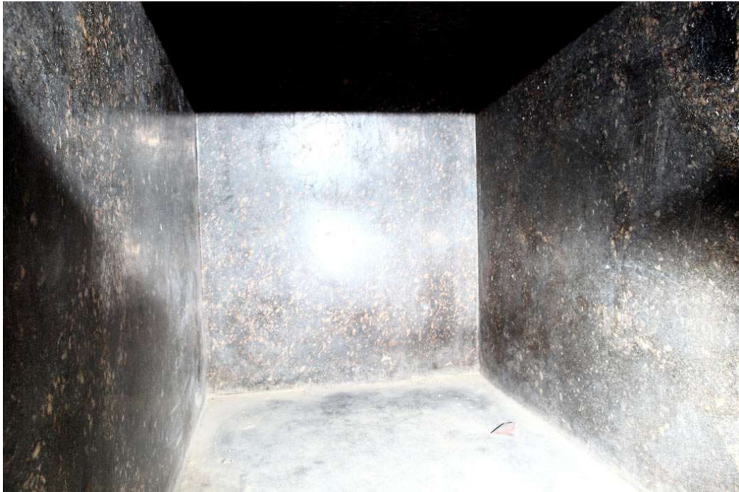
Polished, level, flat surfaces inside the coffers.
