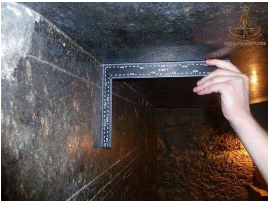
Perfect right angle corners and level surfaces on the inside of the coffers.
